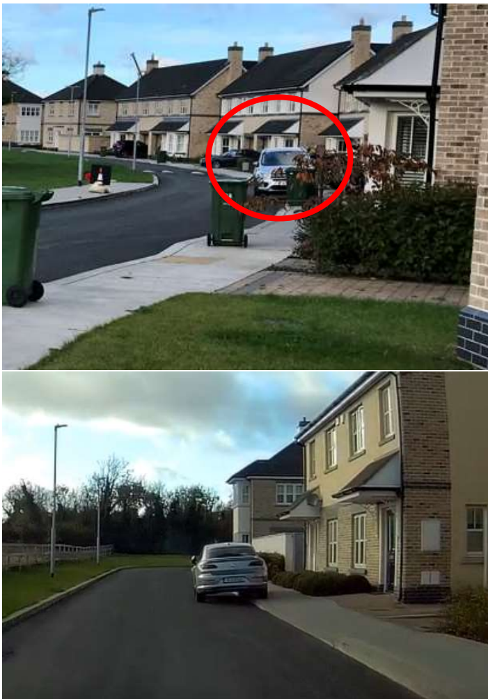
Figure 2.2.1 Examples of cars parallel-parked straddling the footpath in the already constructed part of the estate.
